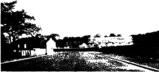
Fig. 2.—Modern Bridge Replacing Above.
